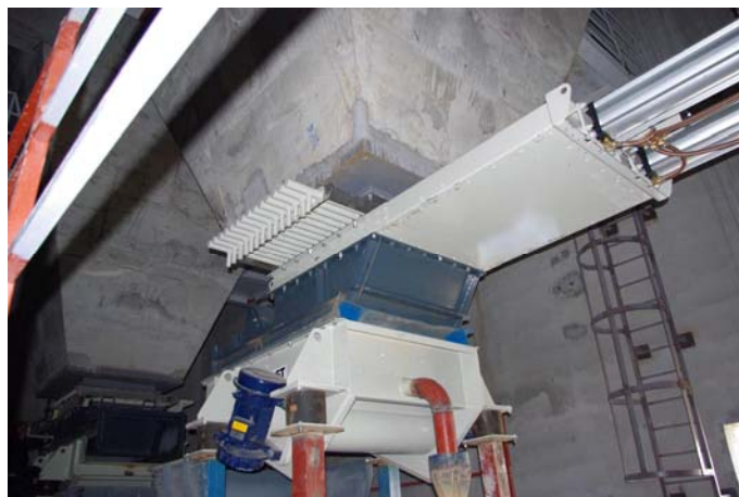
36. picture – Bottom ash silo discharge with vibration feeder – Obrenovac, Serbia
