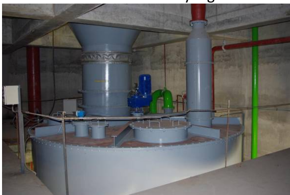
26. picture – Top of conditioner tank Obrenovac, Serbia
