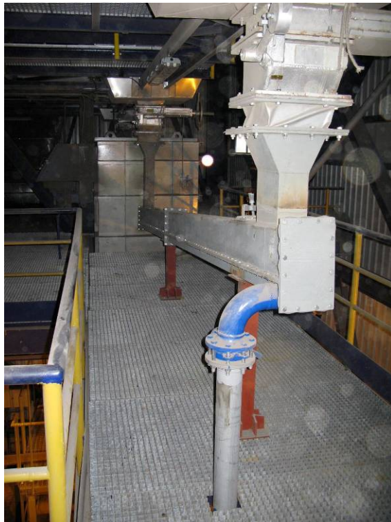
14. picture - Collecting airslides under the ESP – Kolubara, Serbia
