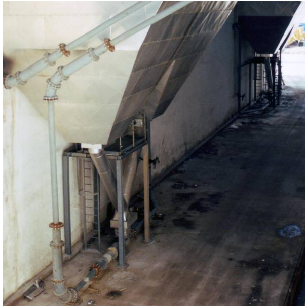
21. picture – Boiler ash conveying with pneumatic jet pump - Agios Dimitrios, Greece
