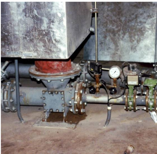
18. picture – Boiler ash conveying with pneumatic jet pump – Steyrermühl, Austria
