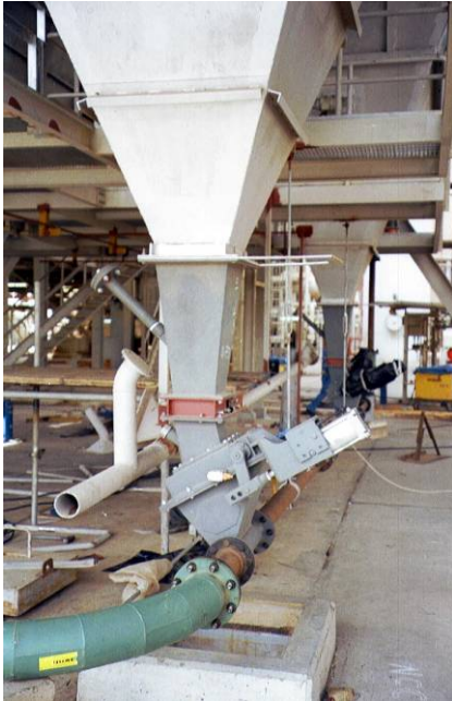
16. picture - Vacuum system under ESP for oil ash - Shoaiba, Saudi Arabia
