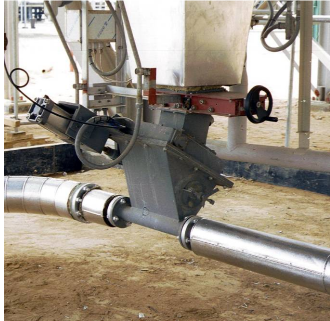
17. picture - Vacuum system under ESP for oil ash - Shoaiba, Saudi Arabia
