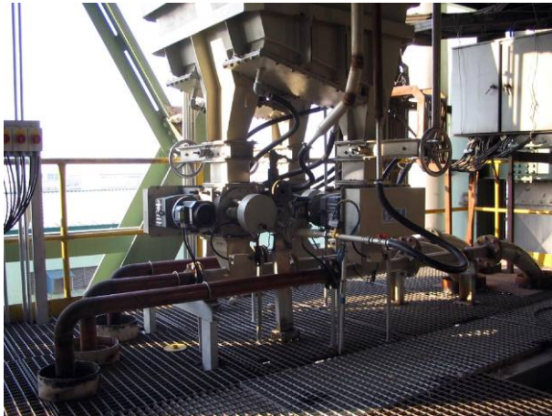
23. picture - Limestone feeding with rotary feeder & feeding shoe into CFB combustion chamber – Chang Shu, China
