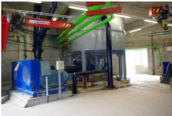
27. picture – Conditioner tank & recirculation pump Obrenovac, Serbia
