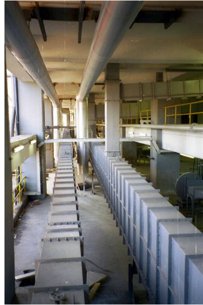
2. picture – Fly ash collection with airslides under ESP – Agios Dimitrios, Greece
