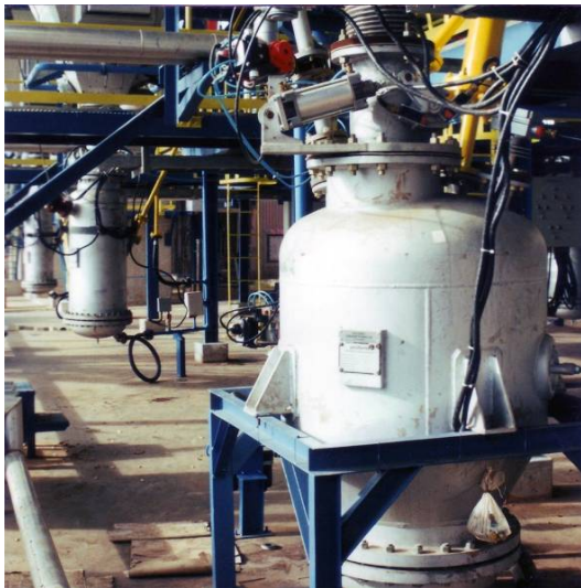
5. picture – Pressure vessel under ESP hoppers – Banjarmasin, Indonesia
