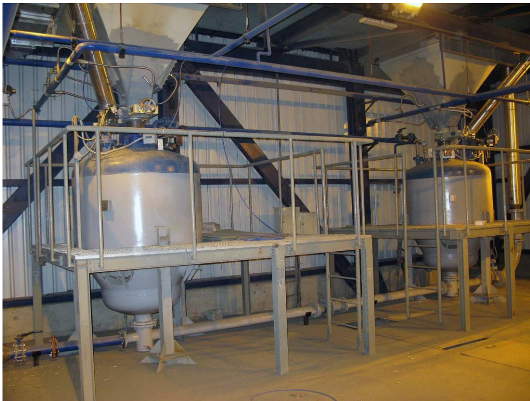
15. picture – Coupled vessels under the ESP – Kolubara, Serbia
