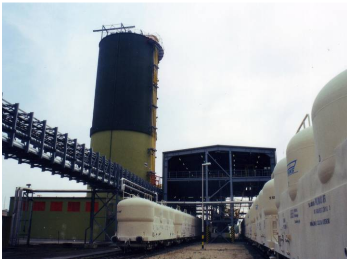
38. picture - Limestone wagon-unloading & storage silo – Mátra, Hungary
