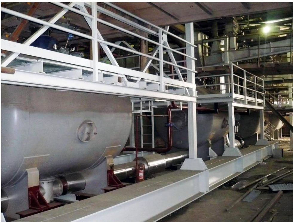
13. picture – Coupled vessels under the ESP – Obrenovac, Serbia
