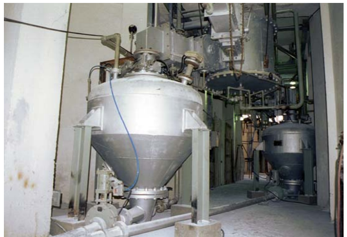
6. picture – Alumina dust pneumatic conveying vessels - India
