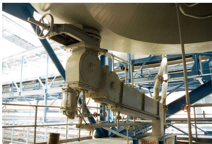
31. picture – Fly ash hopper fluid discharge system – Suralaya, Indonesia
