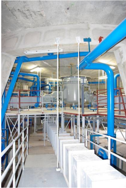
1. picture – Airslide distribution under fly ash silos - Obrenovac, Serbia
