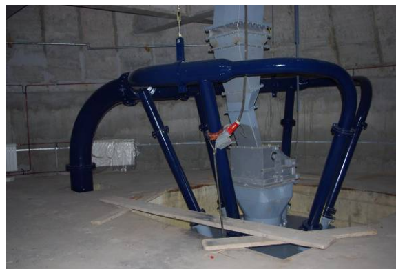
25. picture – Branching pipe & top of premixer Obrenovac, Serbia
