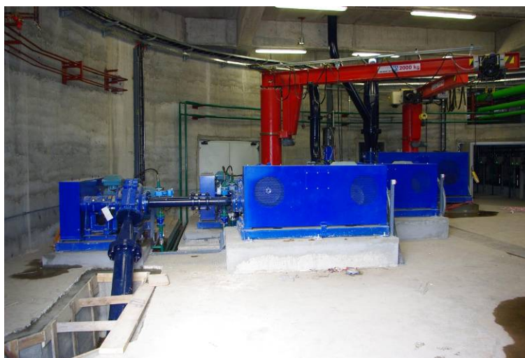
28. picture – Long distance slurry pumps – Obrenovac, Serbia
