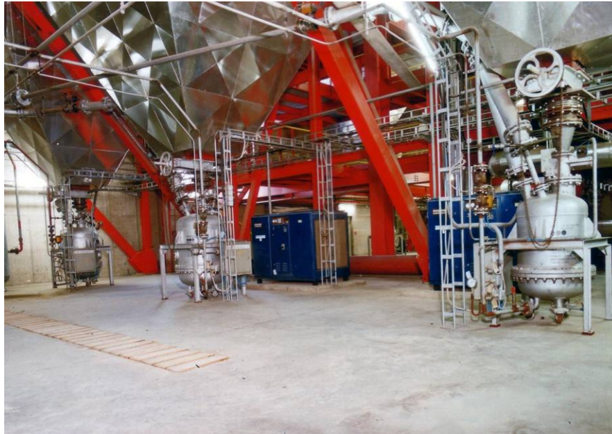
7. picture - Pressure vessel under ESP hoppers – Leykam Gratkorn, Austria
